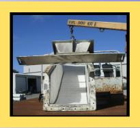
New tiles are cut to size and installed. Wear resist covers tile edges and untiled sections.
