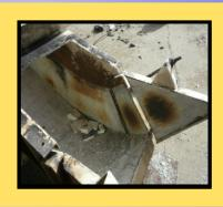
Tiles are removed and the substrate repaired and then blasted.
